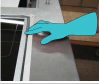
9. Examine the silicone carefully and cut out any bubbles. Fill in any holes with silicone and smooth out the surface again.
